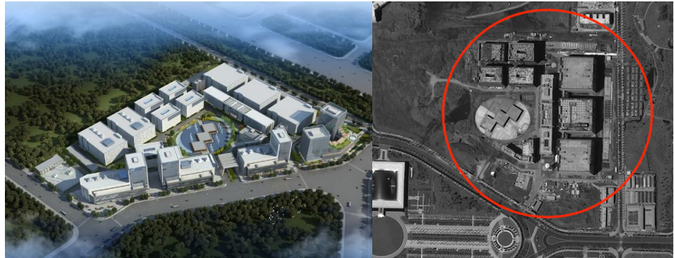
Figure 16: Data Valley concept art (left). Current construction progress (right).
