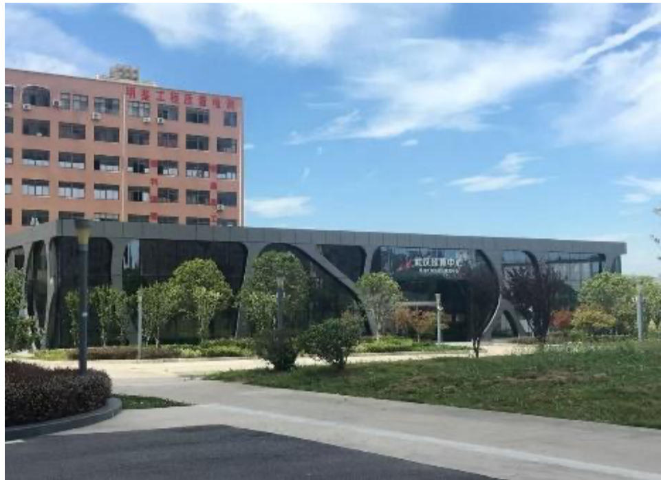
Figure 15: The Supercomputing and Big Data Center, south of the NCC
